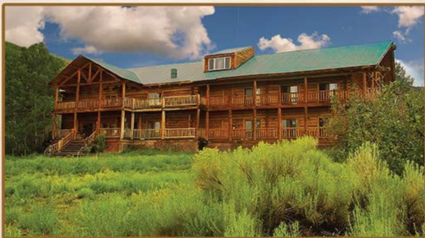
Primary Structure Exterior
