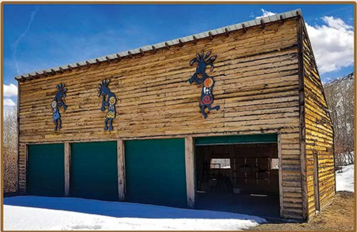
4-Bay Garage / Vocational Education Facility
