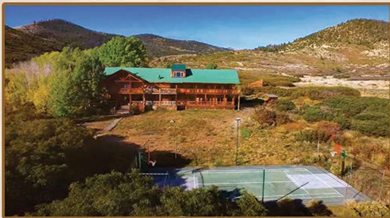
Primary Structure Exterior & Sport Court
