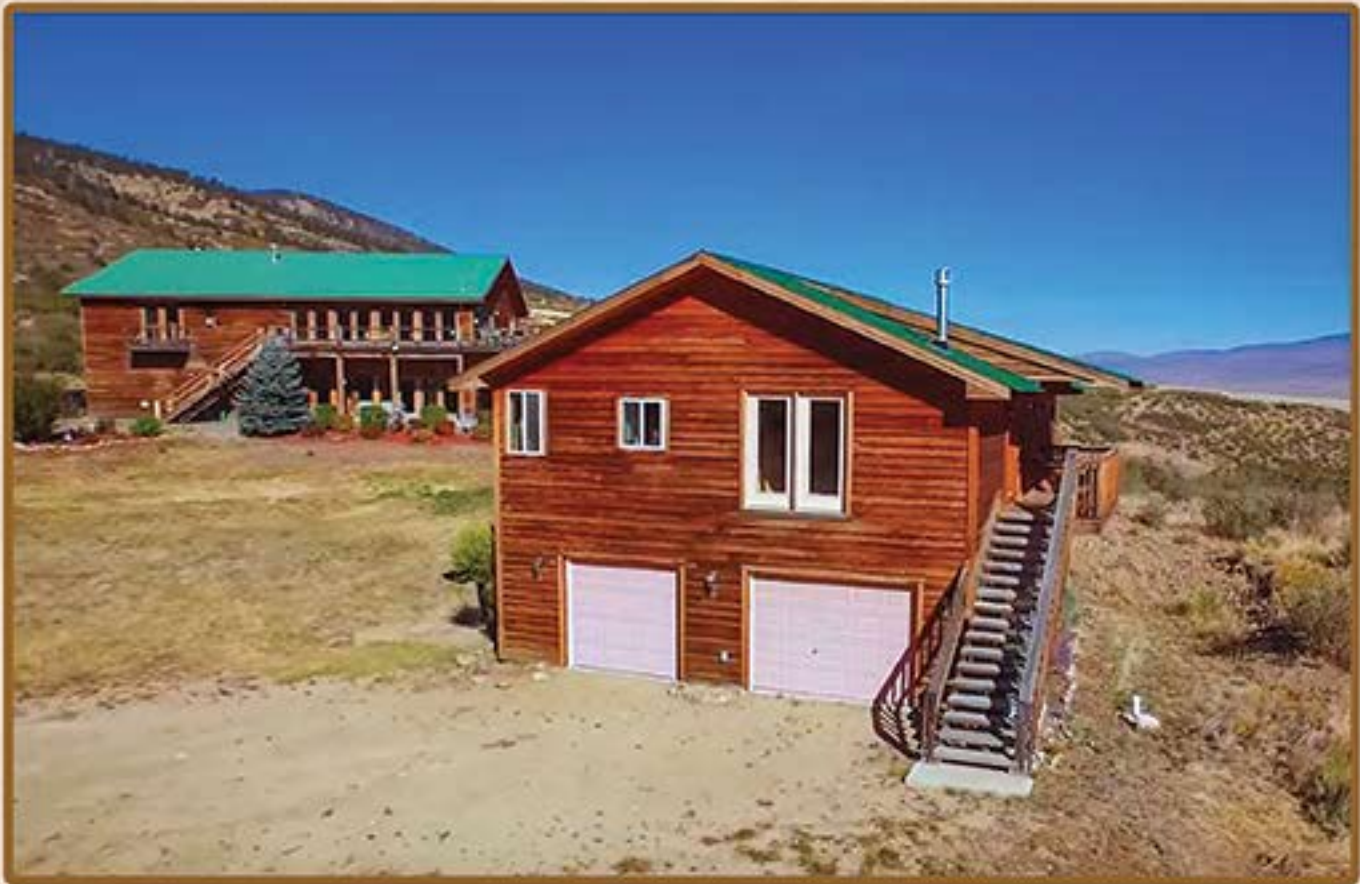
Permanent Housing - Physical Fitness Center & Locker Rooms w/8 Showers, Toilets & Lavatories
